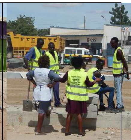
Walk show sensitization at road construction site
