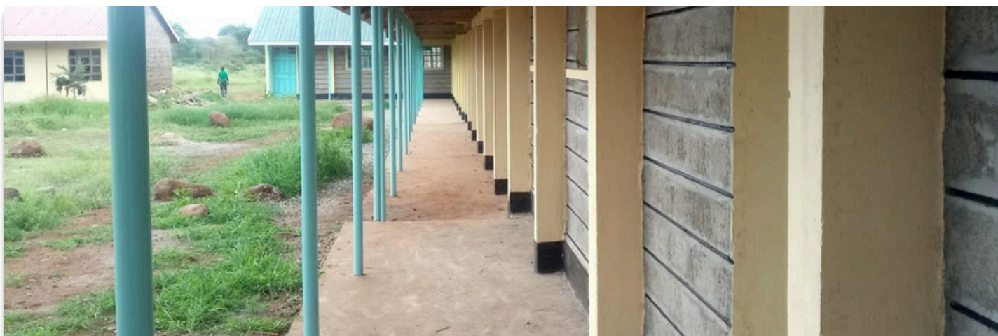
Part of the front pictorial view of the 8No. Classroom block constructed
