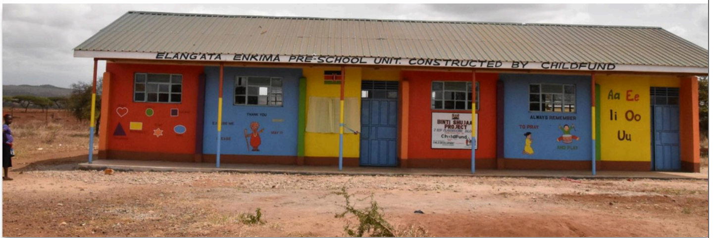
Front view of the ECD Centre constructed
