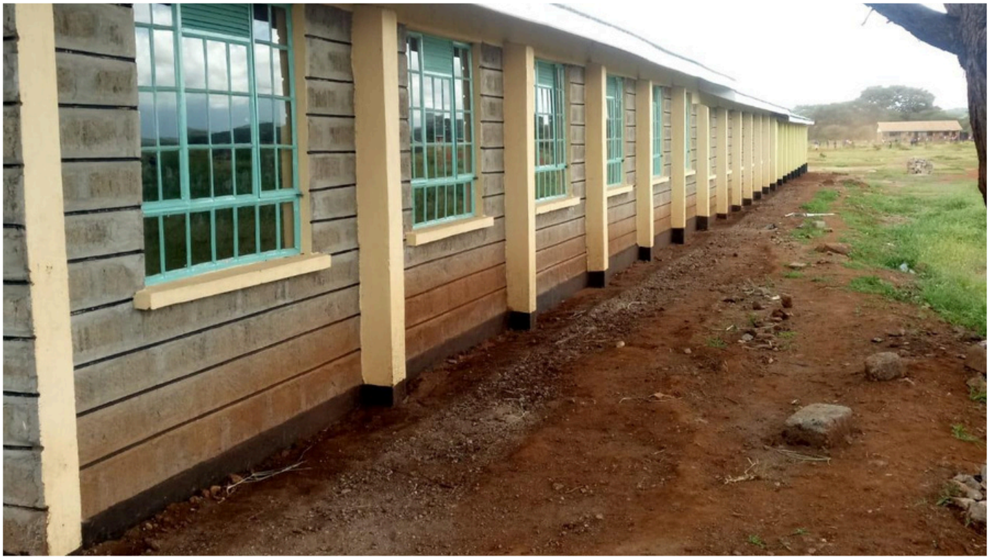
Rear pictorial view of the 8No. classroom block
